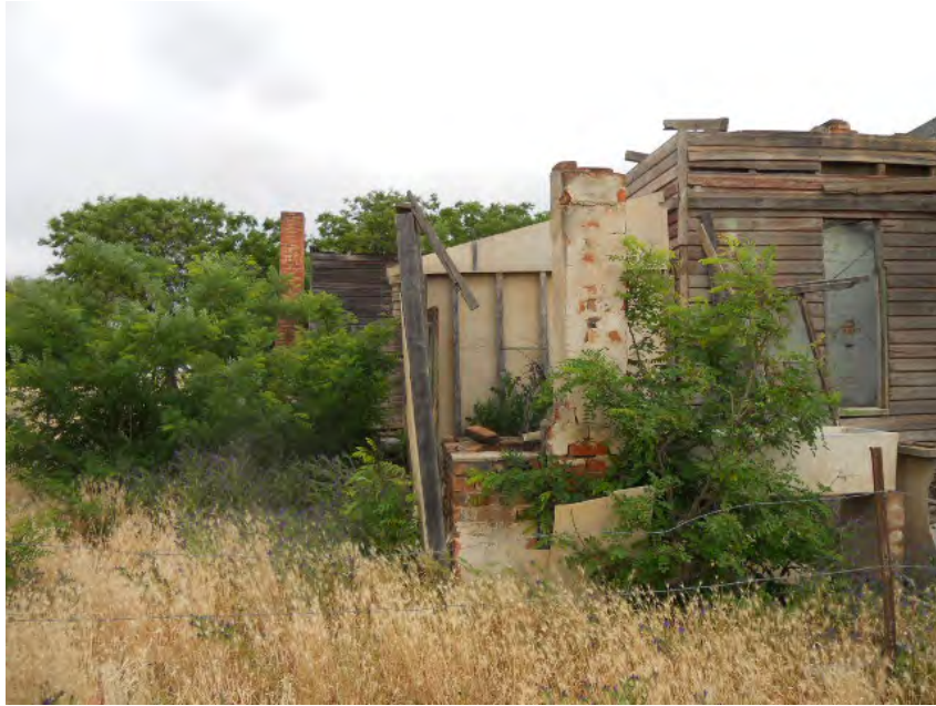
Plate 3.29: The use of fibrolite cladding on the laundry at the eastern end of the building indicates that it was constructed after 1917.
