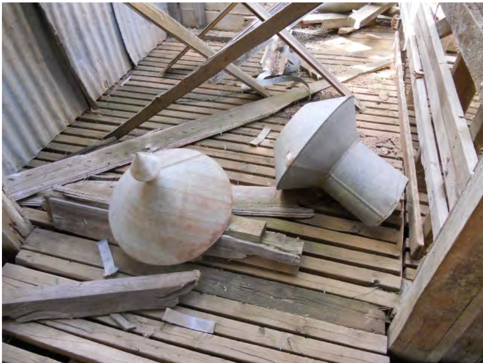
Plate 3.9: Galvanised vents inside the former catching pens.
