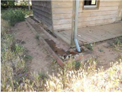
Plates 3.15 & 3.16: Some conservation works have been undertaken on the building with new guttering & downpipes leading to brick drains.
