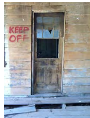
Plates 3.19 & 3.20: The front (left) & back (above) doors of the 1898 teacher's house.
