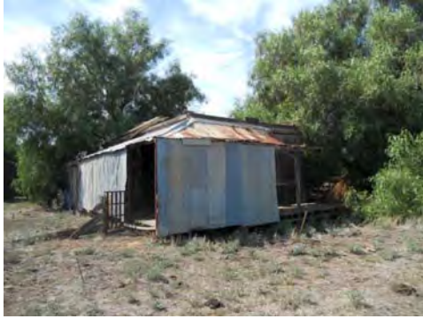
Plate 3.5: Northwestern corner of the former school building.
