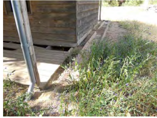
Plates 3.15 & 3.16: Some conservation works have been undertaken on the building with new guttering & downpipes leading to brick drains.
